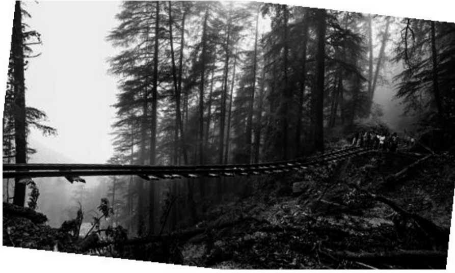
The damaged Shimla-Kalka railway track following a landslide in Shimla on Monday; (below) The Doon Defence College building collapses near Dehradun
